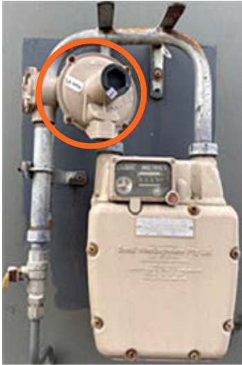
Figure 6 – Gas Vented Regulator
